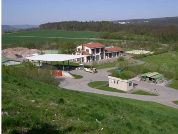
Overview of an Entrance Area
