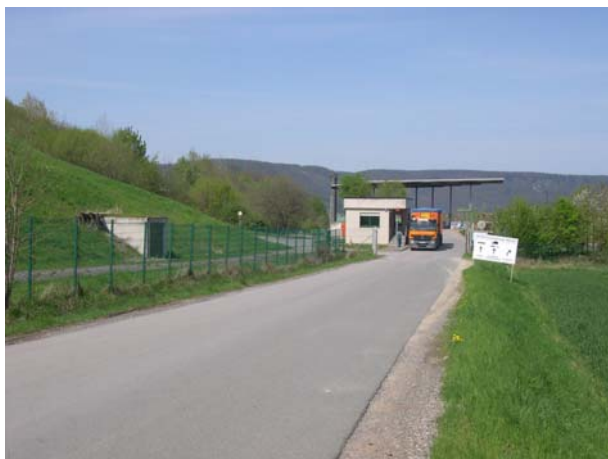
Access Road, Gate and Fence
