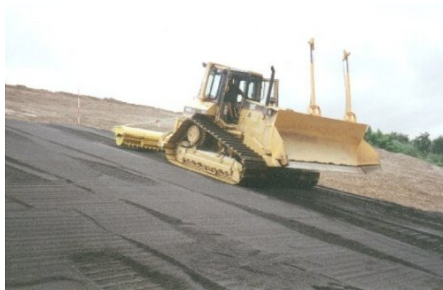
Construction of a Capillary Barrier
