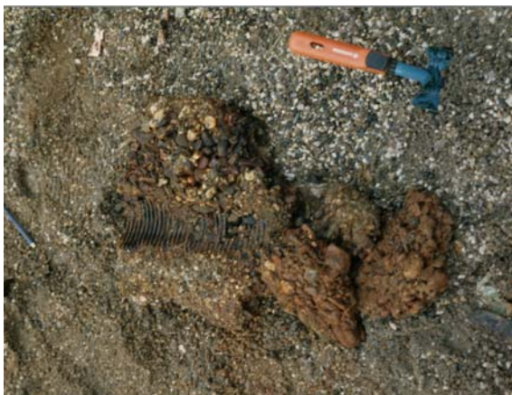
Landfill Geldern-Pont - Detail of drainage material around the drain pipe
