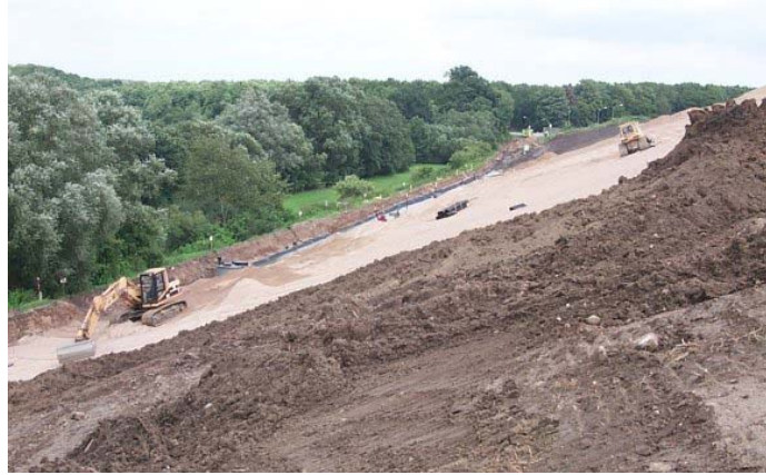
Construction of a Drainage Layer
