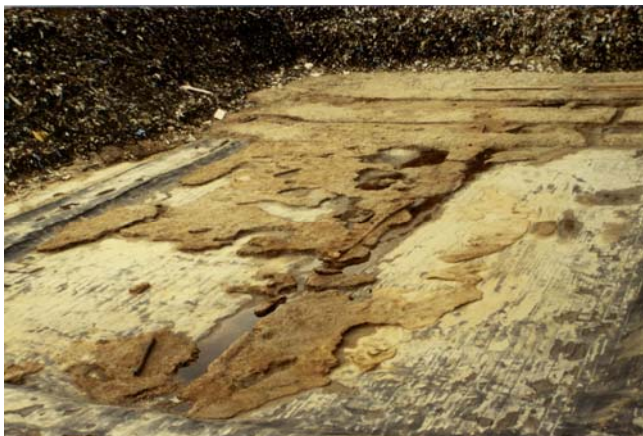
Landfill Geldern-Pont - Overview of the excavated drainage layer
